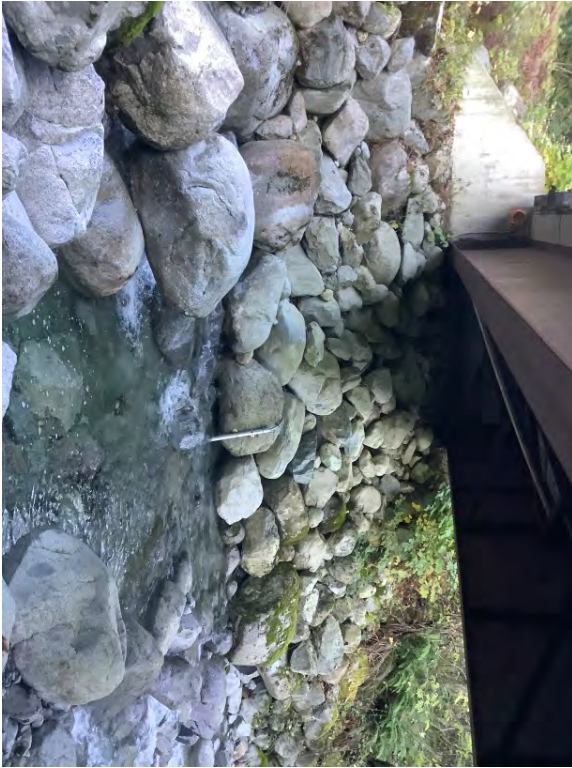
Left Bank Abutment when facing downstream
